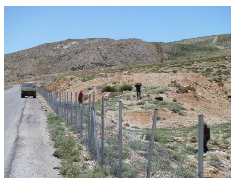
Figure 5-5. Full site fencing with wire fence.
